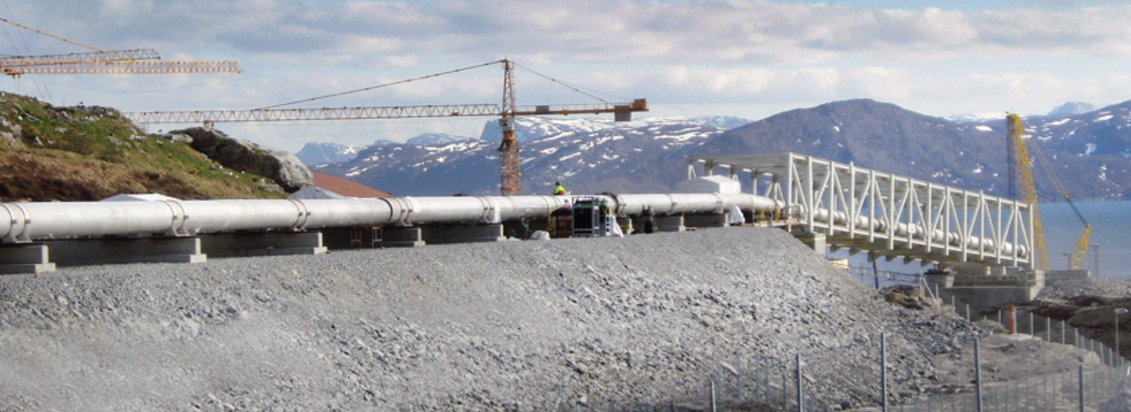
1 600 m of BUTTING pipes – the flareline for the project Snøhvit
